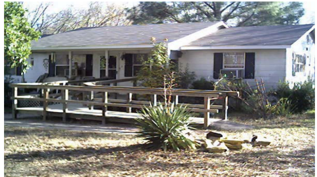
THIS IS ONE OF THE MANY WHEELCHAIR RAMPS THAT ARE BUILT FOR CLIENTS SO THEY CAN EASILY ACCESS THEIR HOMES
